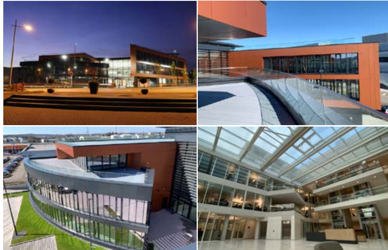
Below: New office building „Beaubourg” [now: Proximus House], Bertrange (L). Project management. Architect Design: Marc Gubbini Architectes | Linster Stupar Architectes. Architect Execution: Architecture et Environnement.
