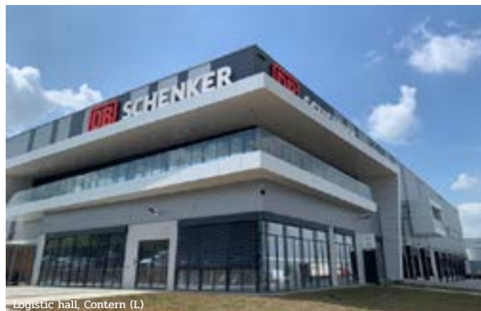
Logistic hall, Contern (L)
